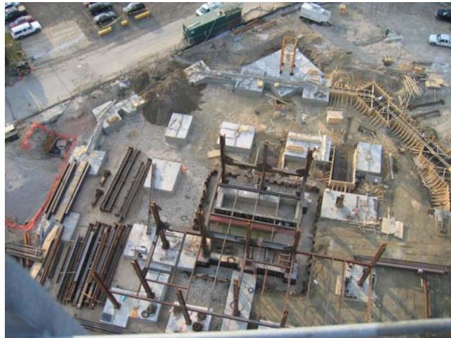
Fig 8 – Aerial view showing poured pile caps and beginning of column erection
