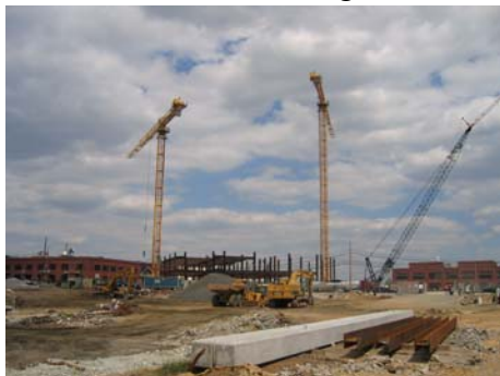
Fig 10 – Tower cranes from afar
