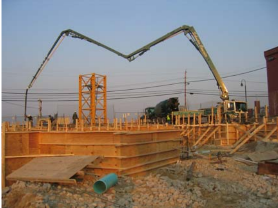
Fig 15 – Concrete Pump during foundation pours
