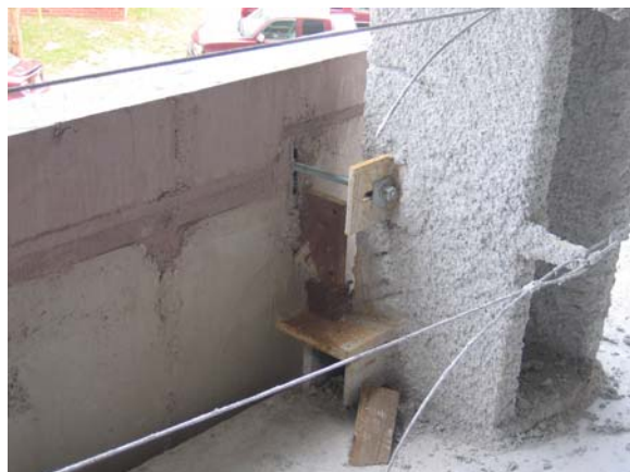
Fig 16 – Precast connections to steel columns
