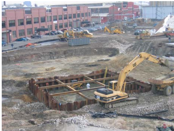
Fig 17 – Shoring for elevator pits
