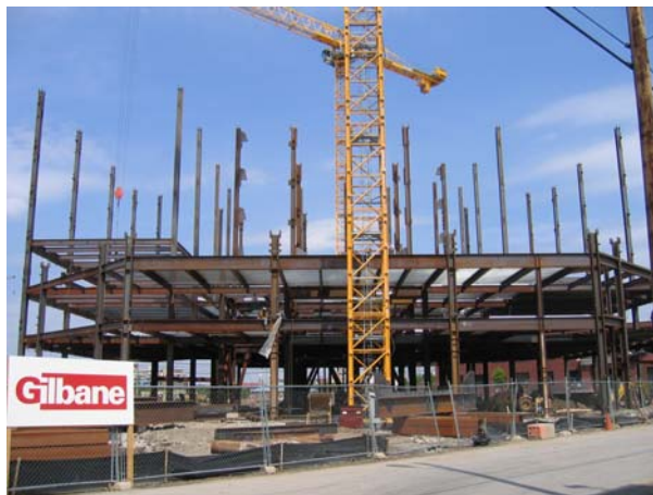
Fig 9 – Steel Column Erection view from Gilbane's field trailer
